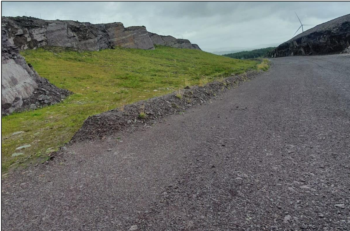
Plate 6-10 Example of reinstatement of roadside verges along the site access track infrastructure classified as Buildings and artificial surfaces (BL3).
